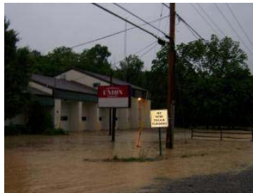
Old Union Firehouse, Boone County Flooding
